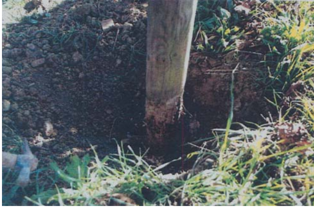
Unimpregnated pole after 4 years, visible damage (Italy)
